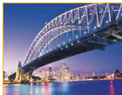
Outdoor Lighting 户外照明
